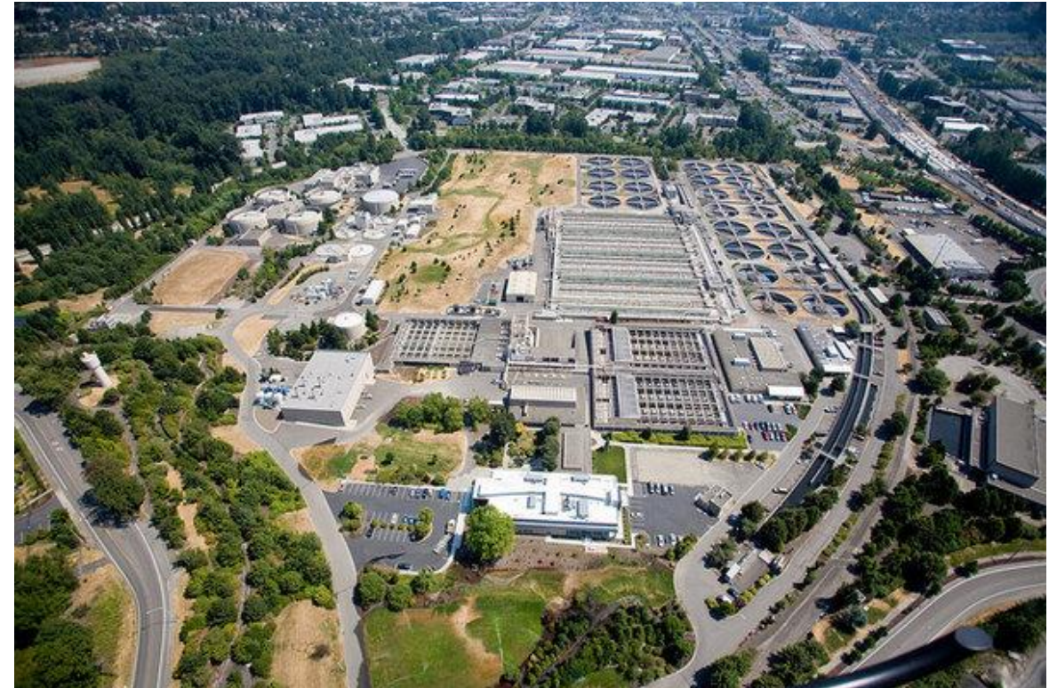
South Treatment Plant
